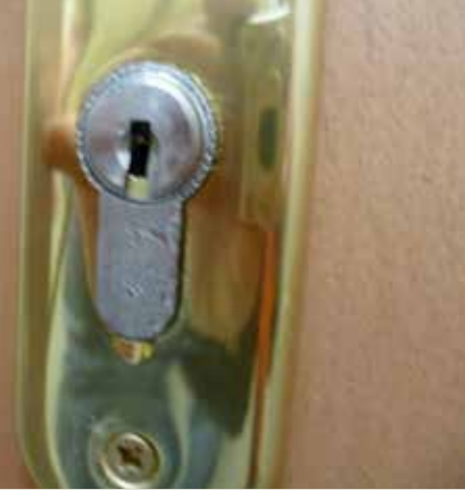
In the laboratory test condensation water formed with a conventional cylinder
