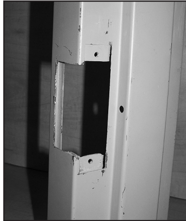
Frame Preparation: Should the frame not be cut out for the ES74F, follow the directions provided on page 2.
