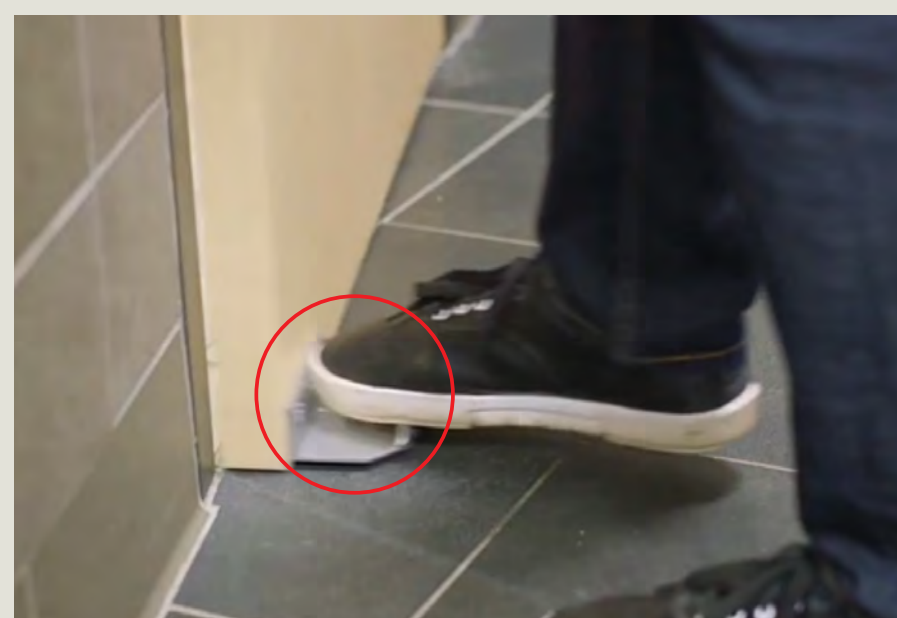
Hands-free access through mechanical doors with a foot pull-handle combined with an overhead door closer
