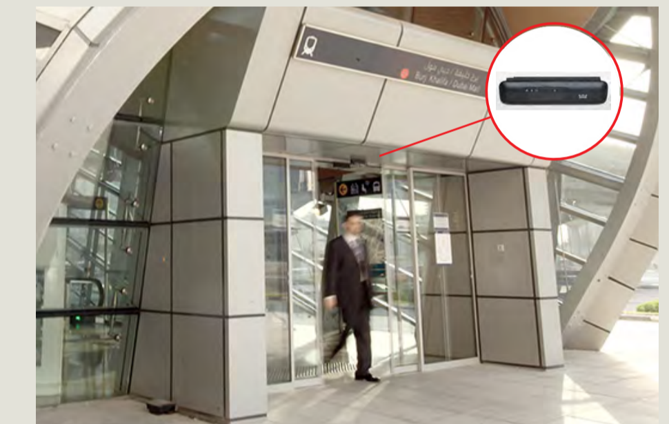
Automatic Sliding door combined with an overhead motion sensor
